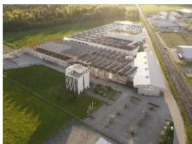
Photo 6: Belimed plant in Sulgen Photo: Belimed
