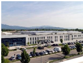
Photo 4: Steelco plant in Riese Pio X Photo: Steelco
