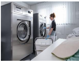
Photo 5: Plenty of space in which to sort and iron laundry: Space planning in the on-premise laundry at the Lavendio retirement home in Melle was the responsibility of Miele – as was equipping the laundry with innovative technology and other accessories. (Photo: Miele)
