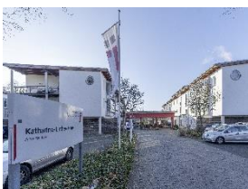
Photo 8: The Katharina Luther care home is part of the protestant Johanneswerk and is located close to the centre of Gütersloh. It offers a home to up to 103 residents. (Photo: Miele)
