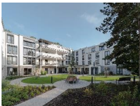
Photo 6: The Lavendio retirement home is located close to the centre of Melle and offers single rooms only to 126 residents. (Photo: Miele)
